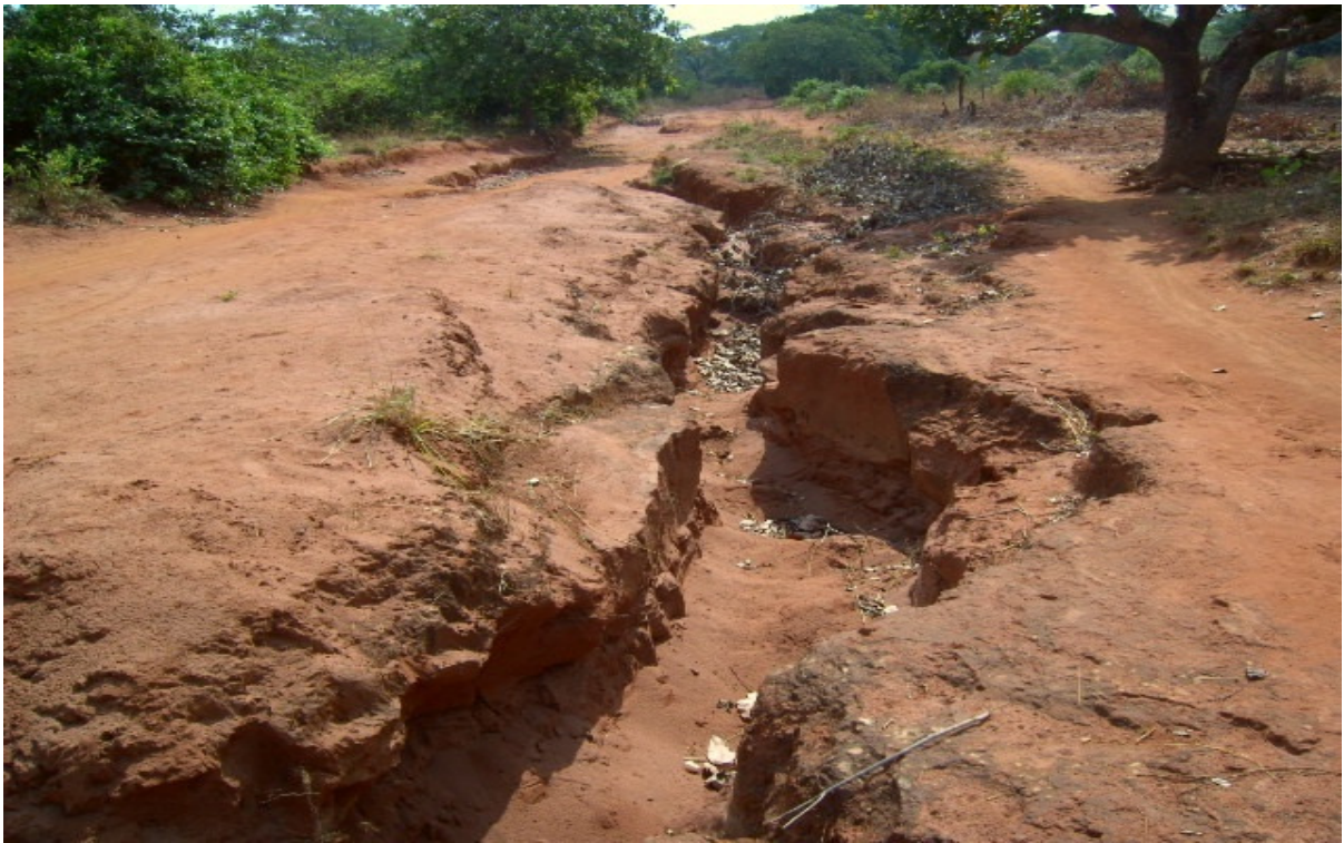
Figure 30 Untarred busy road with erosion channel; Aku to Ozalla road (Photo by Ani U. A. Jan 2009).
