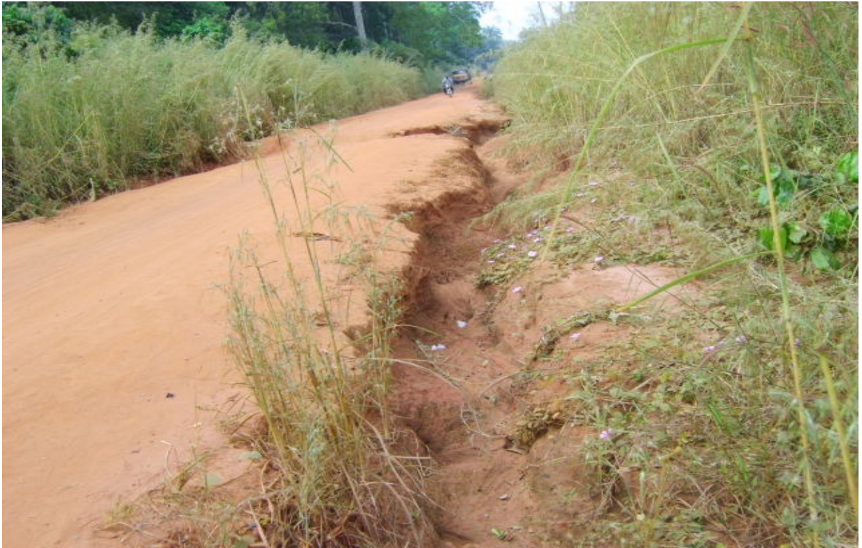
Figure 22 Gully site at Olido near Health Center (Photo by Ani U. A. Jan. 2009)
