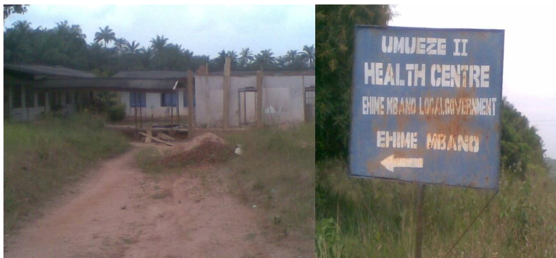
Umueze II Health centre under reconstruction
