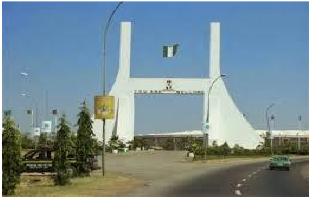
Plate 1: The Entrance City Gate of Abuja
