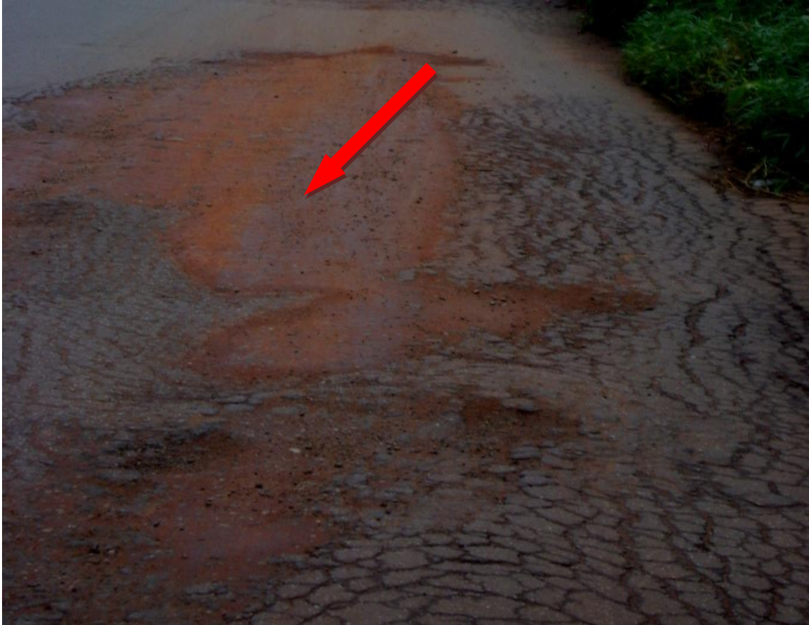
PLATE 7: This picture shows the part of the road where the transverse/perpendicular profile was taken with thin surface coating.
