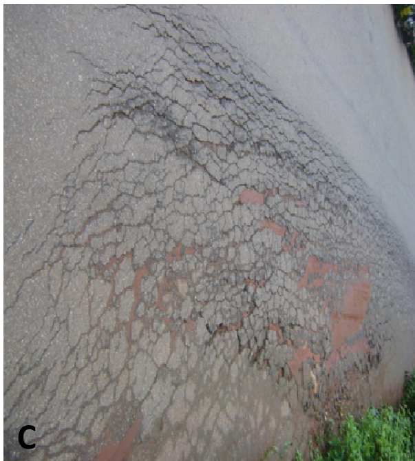
PLATE 1: (A) Failed section of Opoji old road along Opoji ñ Irrua road (B) Pavement surface removal after rehabilitation along Uhiele ñ Opoji road (C) Zoomed section showing very thin coating of the pavement surface (D) Longitudinal view of Uhiele ñ Opoji road with very thin surface coating.
