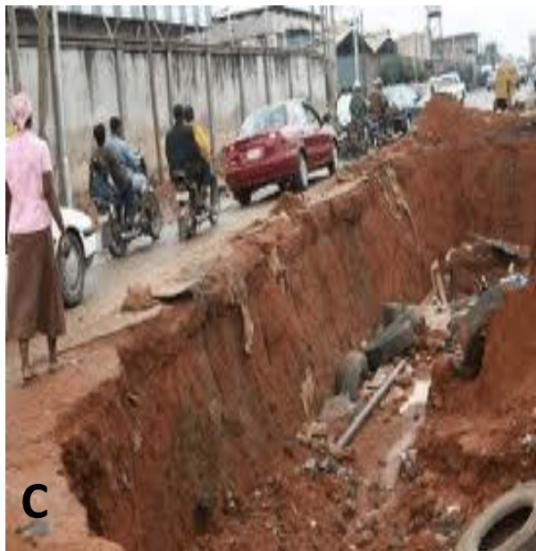
PLATE 2: Major Highways failing before their design age within the state. (A) A Federal highway route in the country (B) and (C) Roads collapsing due to lack of proper drainage system within the state in Benin metropolis (D) Benin ñ Ore road (2010) (Wednesday, 13 July 2011, Nigerian Compass)
