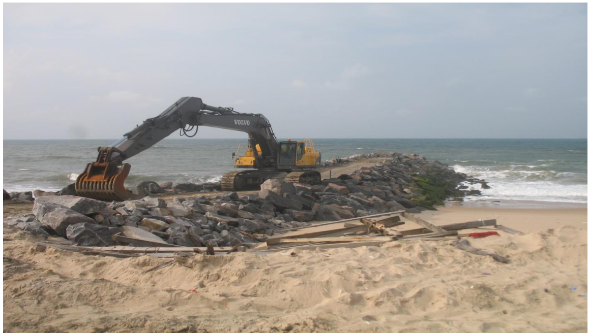
Plate 18: The gigantic rocks used in controlling coastal flooding at the beach (Preventive measure)
