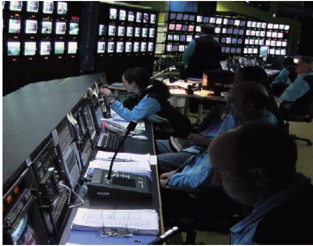
Figure 1.7 Master control room with work stations
