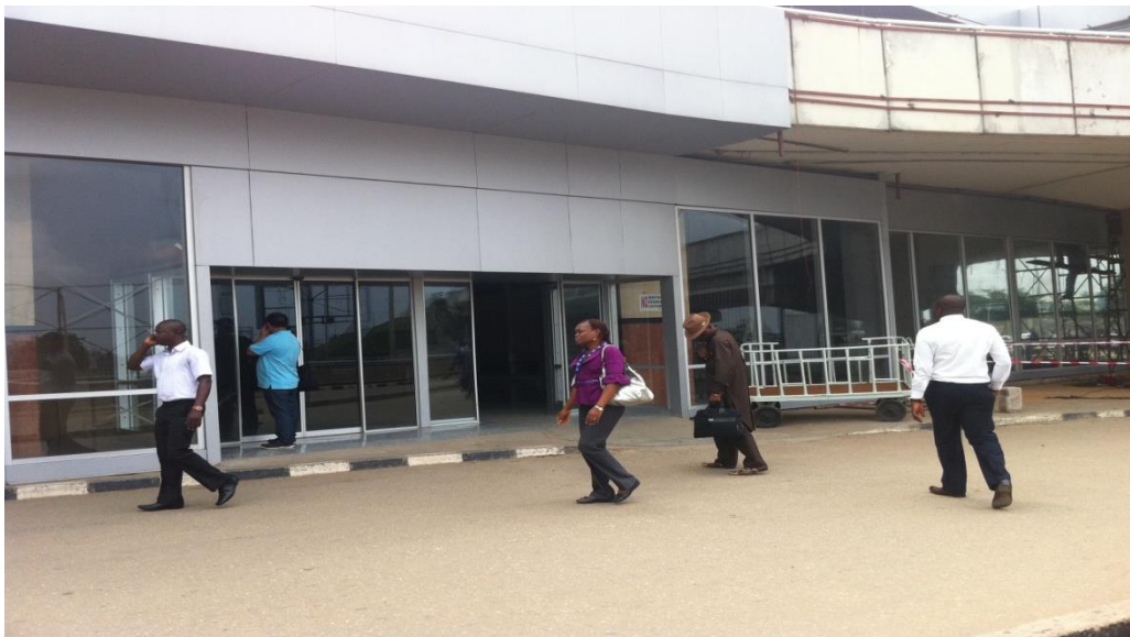
Plate 7: Showing Arrival Hall (Front View) still under remodeling in MMIA.
