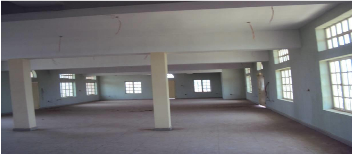
Plate 3.18: Interior view of the first floor multi-purpose Hall .
