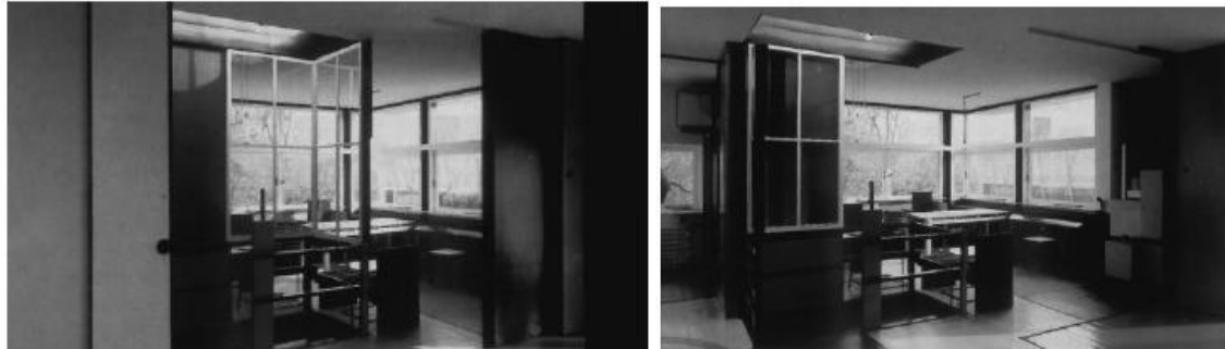
Plate 2.2a and 2.2b: Upper floor of the Schroder house with partitions partially closed (left) and with partitions open (right)
