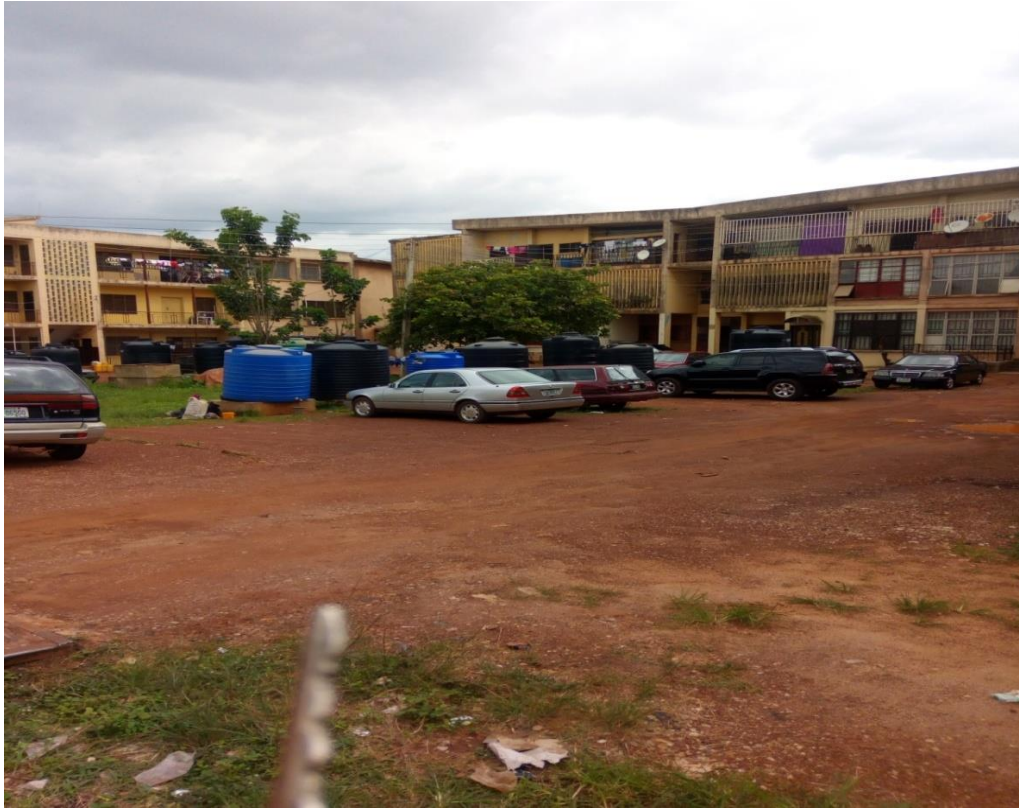
Plate11: Adapted Water Storage and Car Parking on improper designed open space
