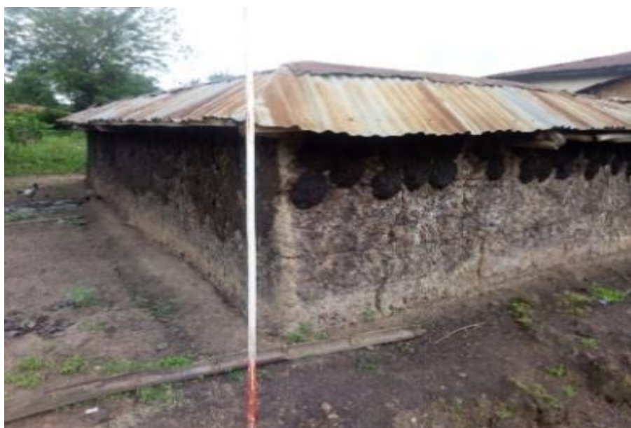
Plate 11: Oguso plastered to a wall.
