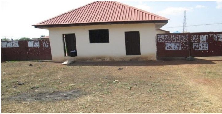
Plate: 27 showing building of National Commission for Museums and Monuments Abakaliki
