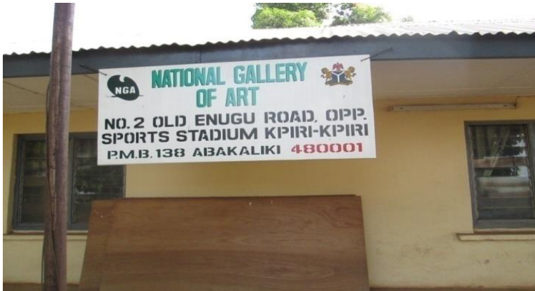
Plate: 29 showing building of National Arts Gallery Abakaliki
