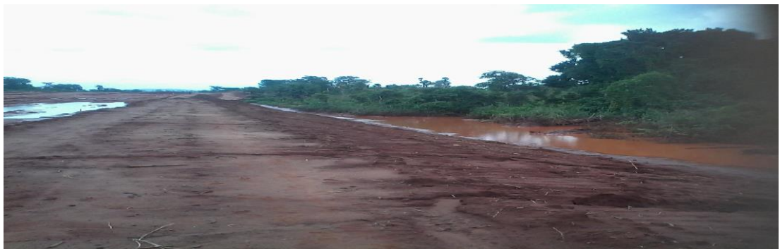
Plate 6: Changes on the Study Area Due to on-going Construction
