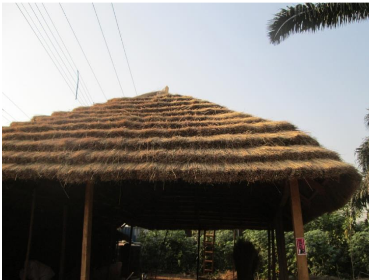
Plate Fifty Four: Showing a thatch roof under construction with ( Imperata cylindrica ).
