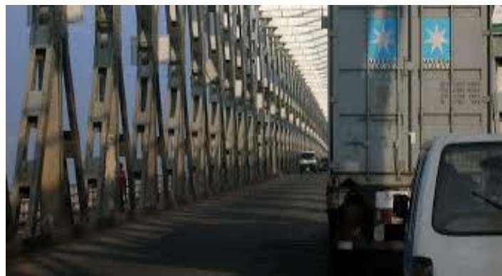
PLATE 1: ONITSHA MAIN BRIDGE
